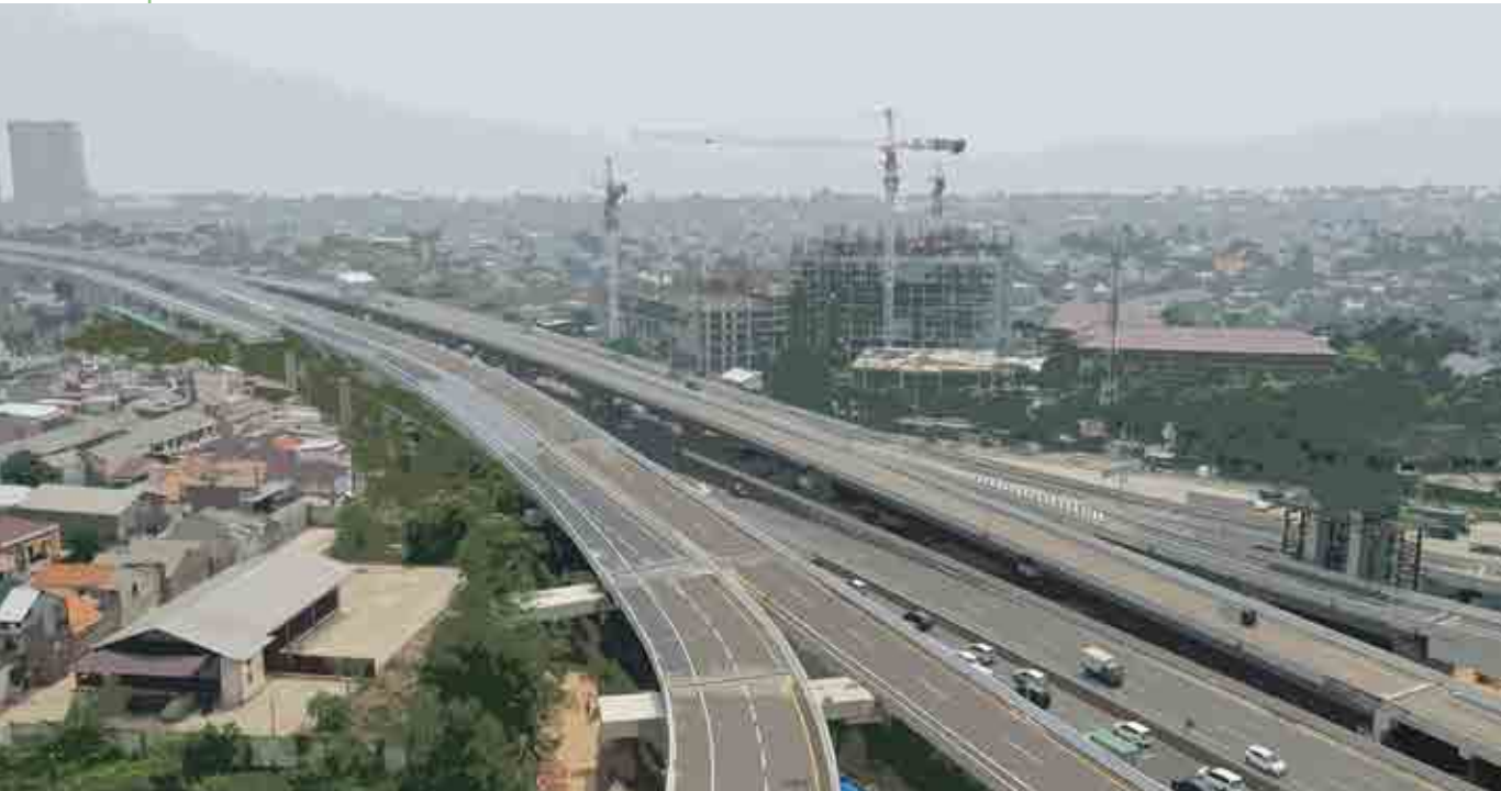
Jalan Tol Jakarta - Cikampek II Elevated / Jakarta - Cikampek II Elevated Toll Road
